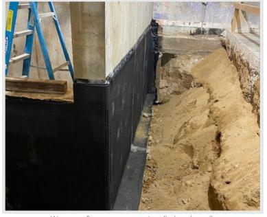
Waterproofing treatment was installed on the walls of the new elevator shaft in the lower-level locker room and multipurpose room addition.
