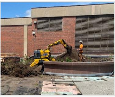
Remote-control robotic equipment is used for demolition work in preparation for the new multipurpose room addition in the courtyard.
