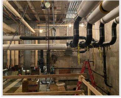
New hot/cold water supply and return piping were installed, which will improve the efficiency and control of the heating and cooling systems throughout the school.
