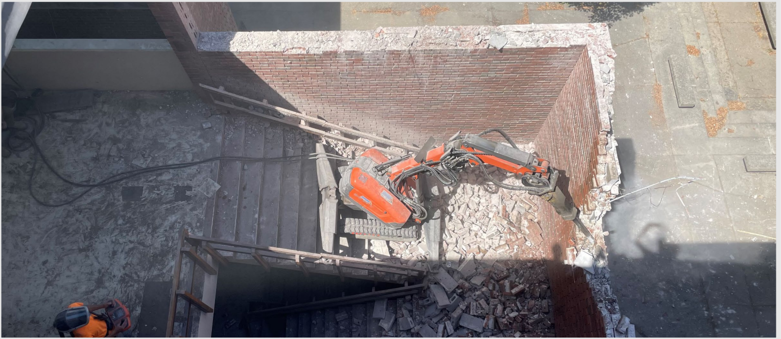
A construction worker used a remote-controlled robot for the demolition of the three-story stairwell and exterior walls in the courtyard area
