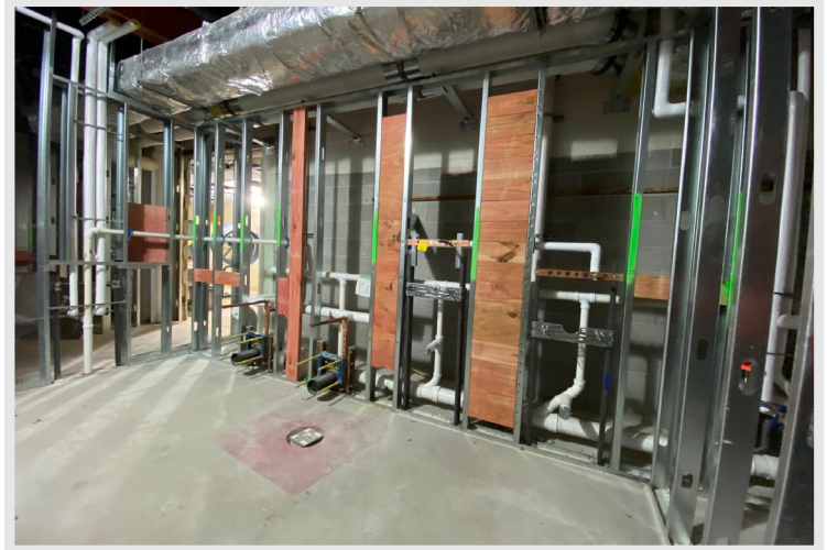
In-wall support blocking and piping have been installed in the bathrooms to provide stability for the partitions and prepare for fixtures
