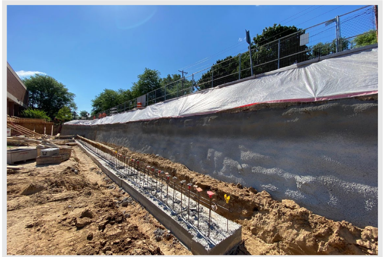
The earth retention system and first concrete footings were installed on the south side of the project site
