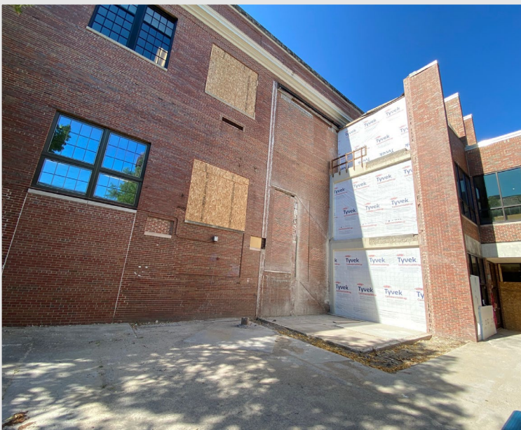
After the stairwell was removed, temporary walls were installed for safety and weather protection
